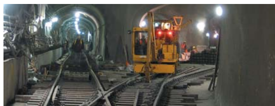
Reconstructed Hudson River PATH tunnels
