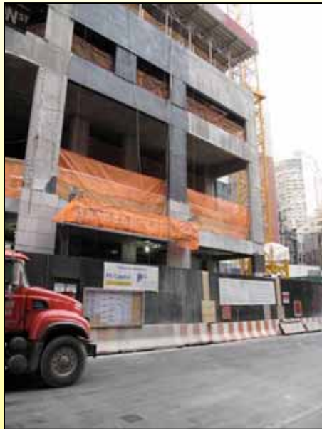
123 Washington Street Site
