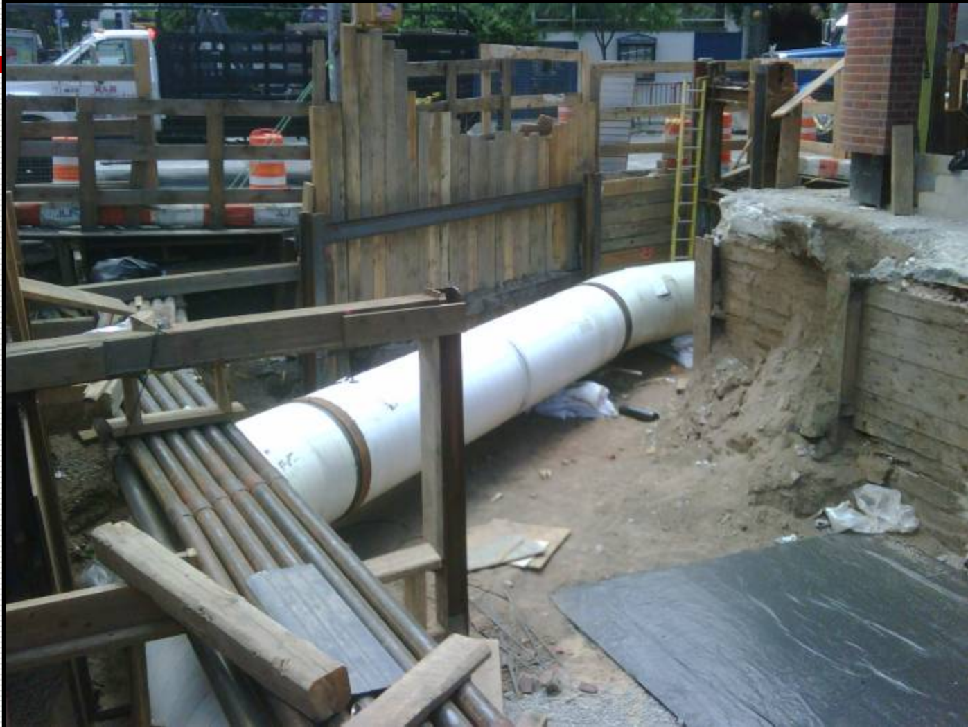
INSTALLATION OF TRUNK WATER MAINS ON HUDSON STREET Project ID: MED596
