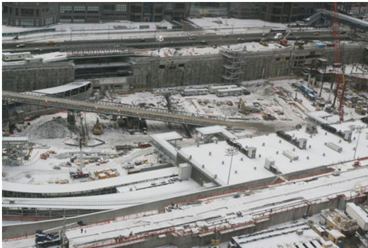
Current construction at the World Trade Center site in Lower Manhattan
